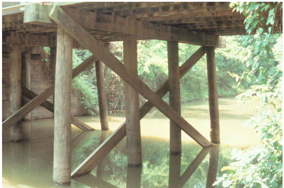
Figure 12.2.39 Timber Bent Columns in Water
