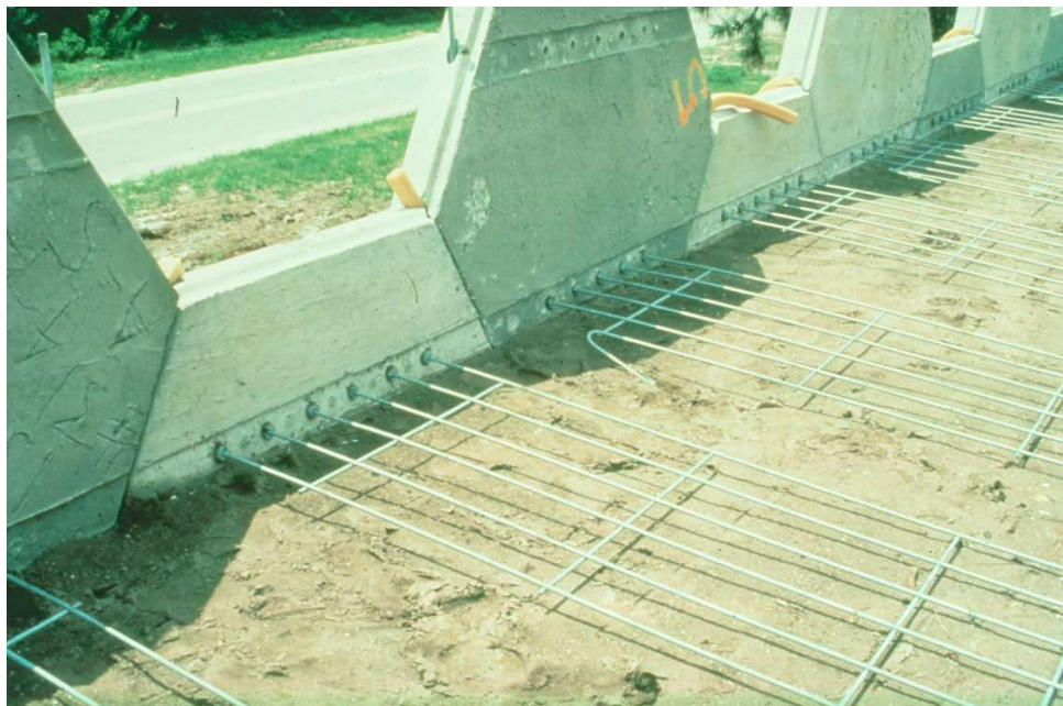
Figure 12.1.10 Mechanically Stabilized Earth Wall Under Construction
