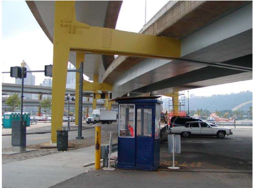
Figure 12.2.51 Fracture Critical Steel Bent
