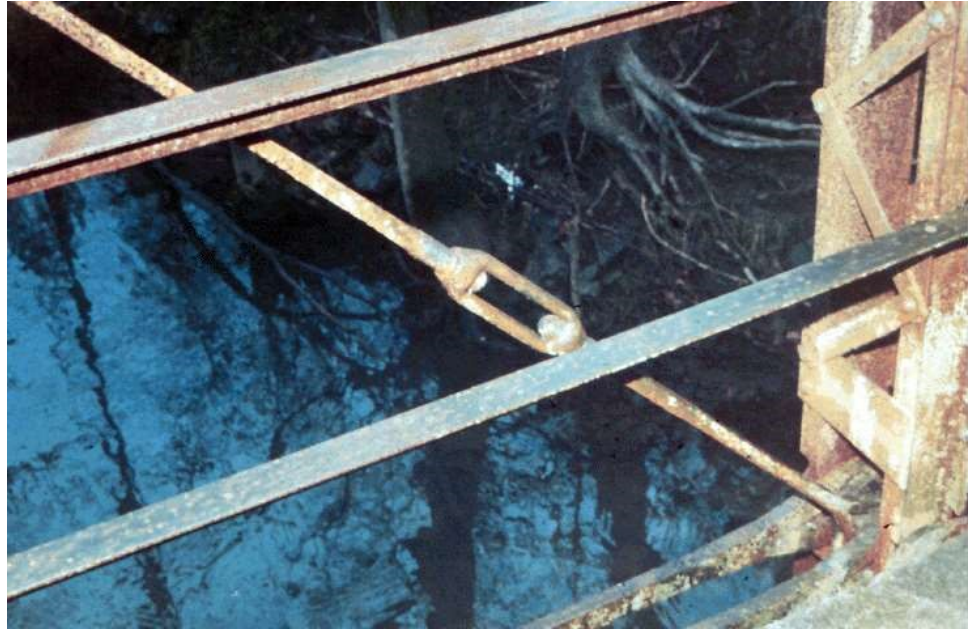
Figure 10.9.28 Turnbuckle on a Truss Diagonal
