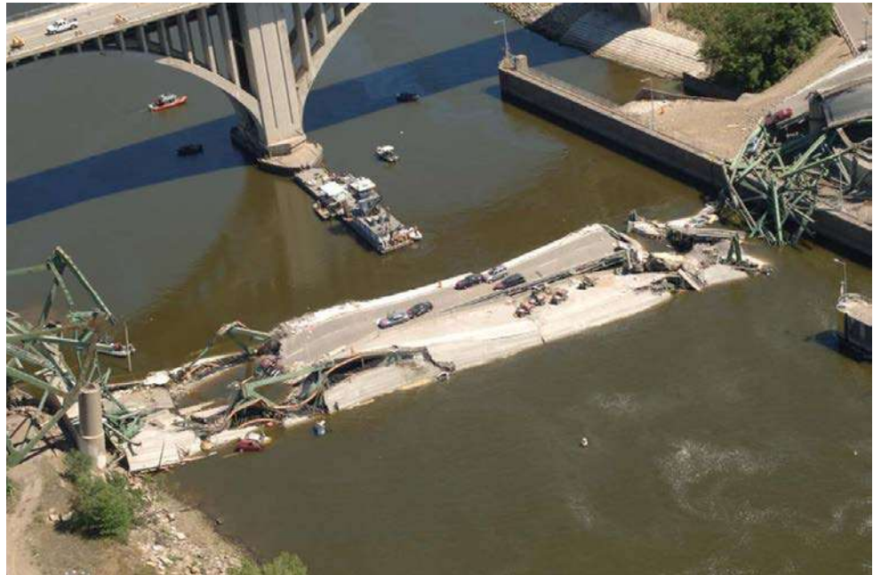
Figure 10.8.34 Collapsed I-35W Mississippi River Bridge
