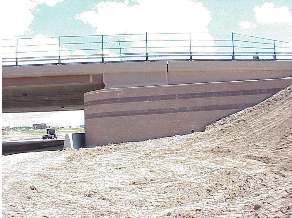
Figure 12.1.12 View of the Founders/Meadows Bridge Supported by GRS Abutments
