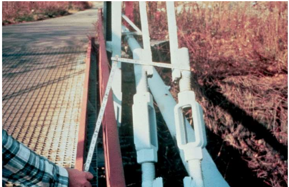
Figure 10.9.29 Welded Repair to Turnbuckles
