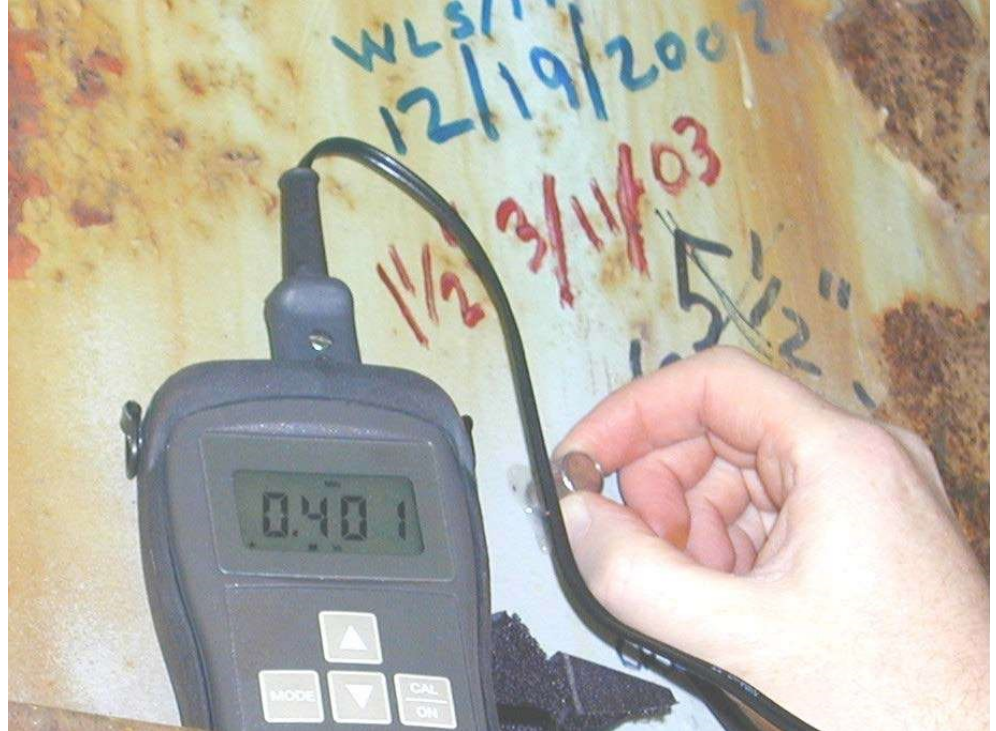
Figure 10.8.19 Inspector Using a D-meter to Measure the Thickness of the Gusset Plate
