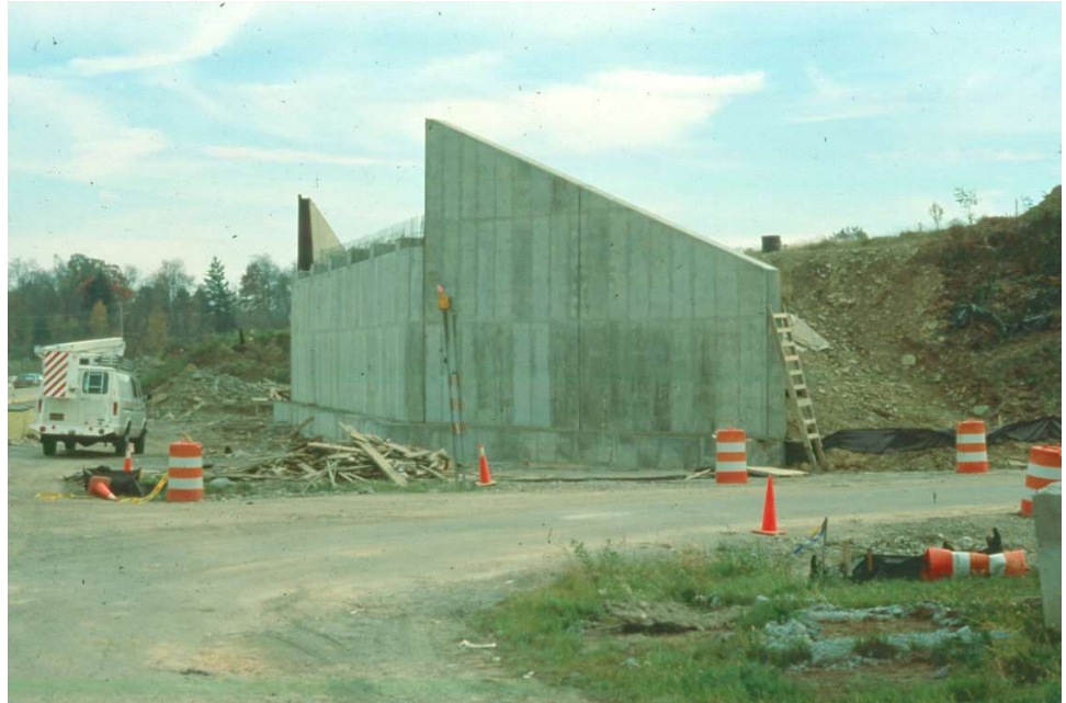
Figure 12.1.14 Reinforced Concrete Cantilever Abutment
