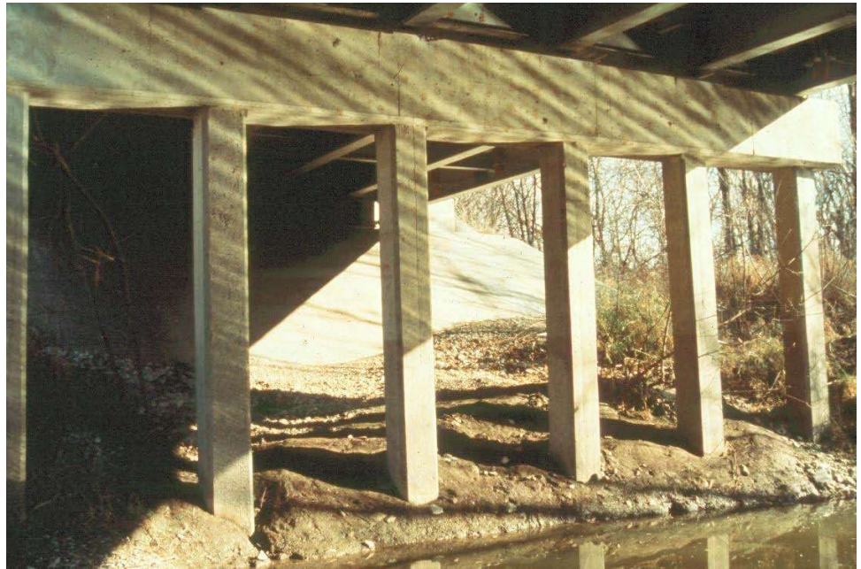
Figure 12.2.9 Concrete Pile Bent
