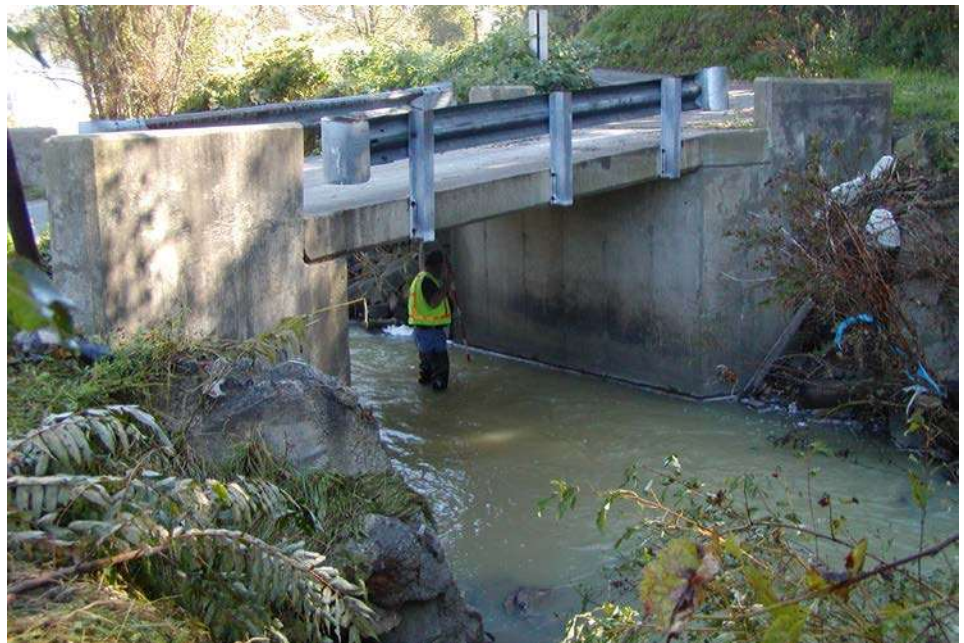
Figure 12.1.51 Inspector Checking for Scour
