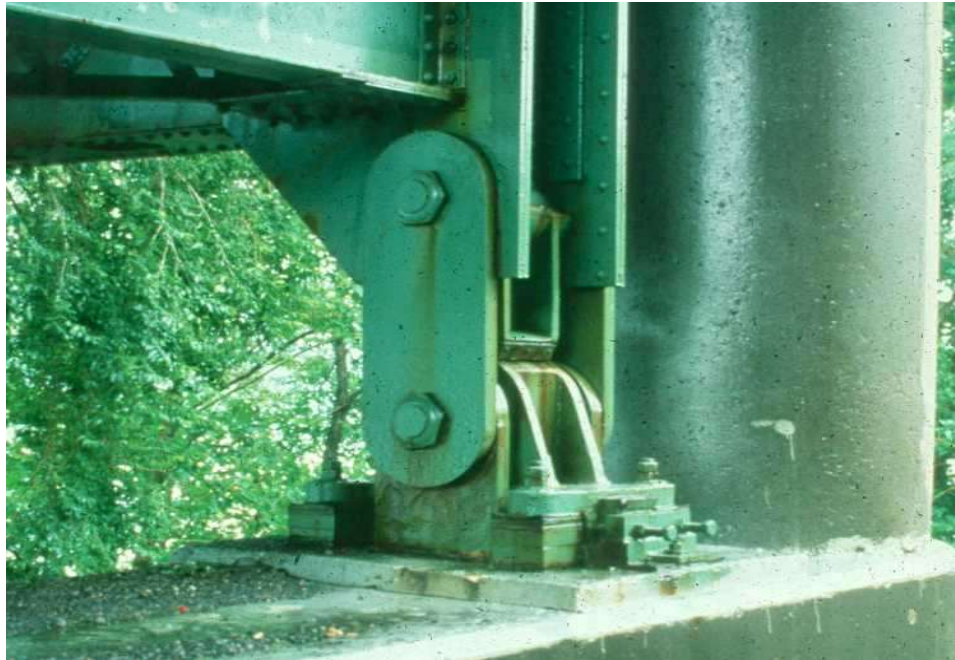
Figure 11.1.19 Pin and Link Bearing
