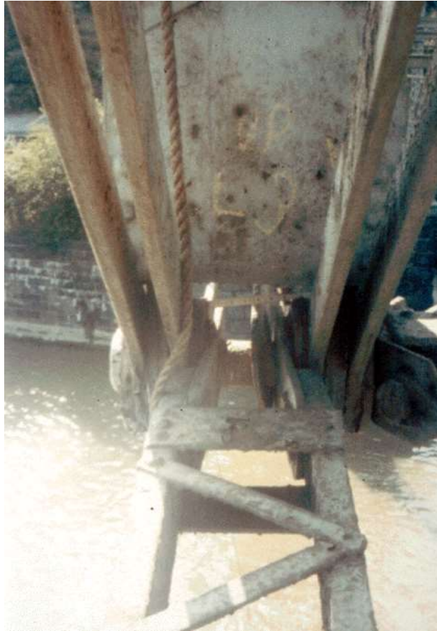
Figure 10.9.15 Loosely Packed Eyebar Connection
