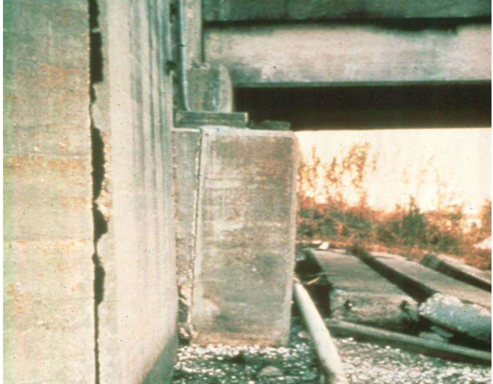
Figure 12.1.47 Rotational Movement at Abutment
