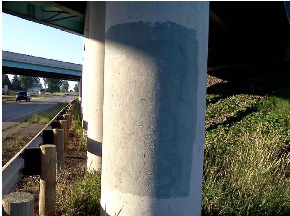
Figure 12.2.50 Repaired Concrete Column Bent
