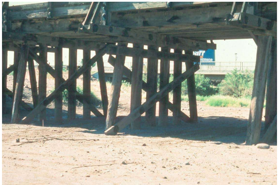
Figure 12.2.16 Timber Pile Bent
