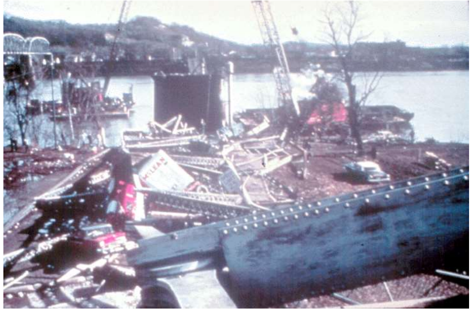
Figure 10.9.5 Collapsed Silver Bridge
