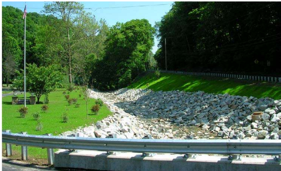
Figure 13.1.9 Crushed Stone Riprap
