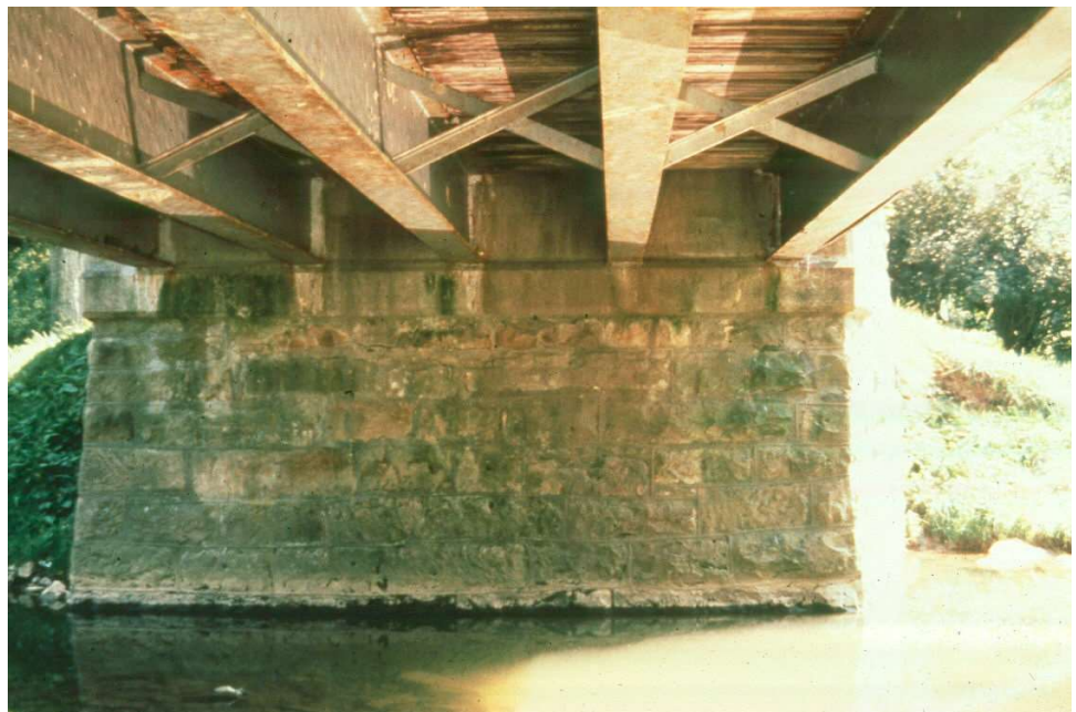
Figure 12.1.15 Stone Masonry Gravity Abutment
