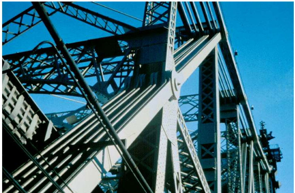
Figure 10.9.2 Eyebare Cantilevered Truss Bridge (Queensboro Bridge, NYC)
