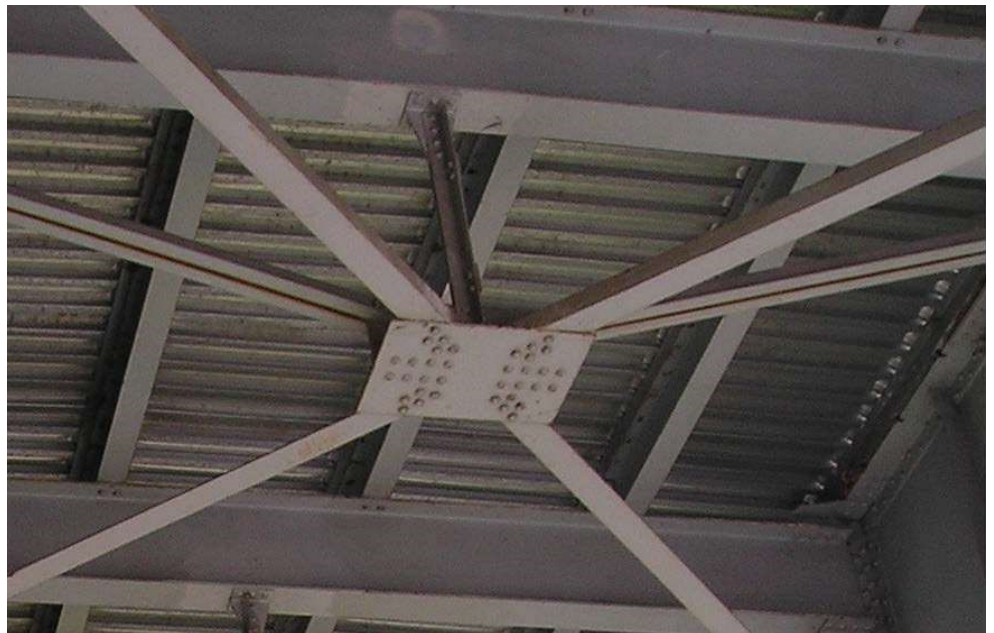
Figure 10.8.15 Gusset Plate Connecting Secondary (Bracing) Members on a Steel Two-Girder Bridge
