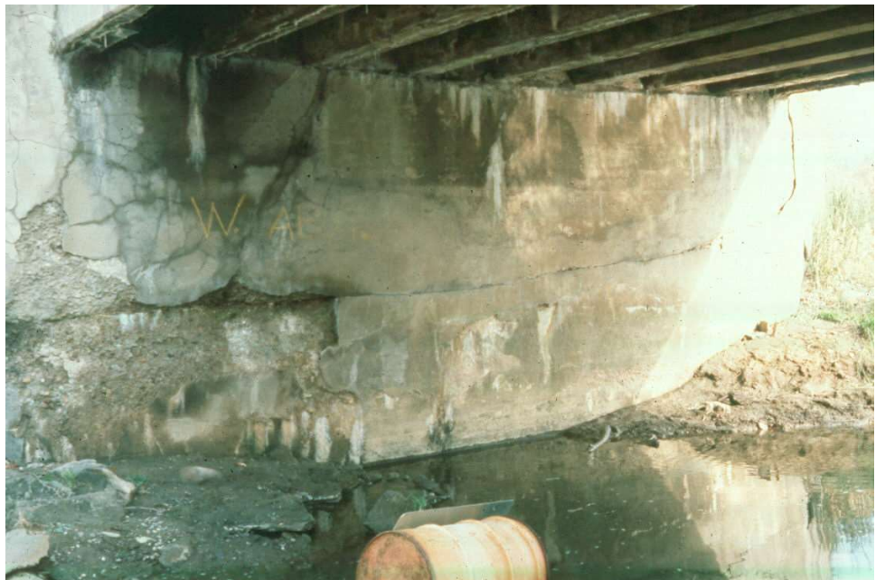
Figure 12.1.13 Plain Unreinforced Concrete Gravity Abutment
