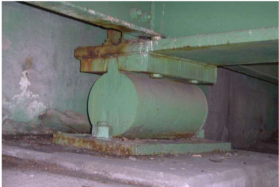
Figure 11.1.7 Single Roller Bearing
