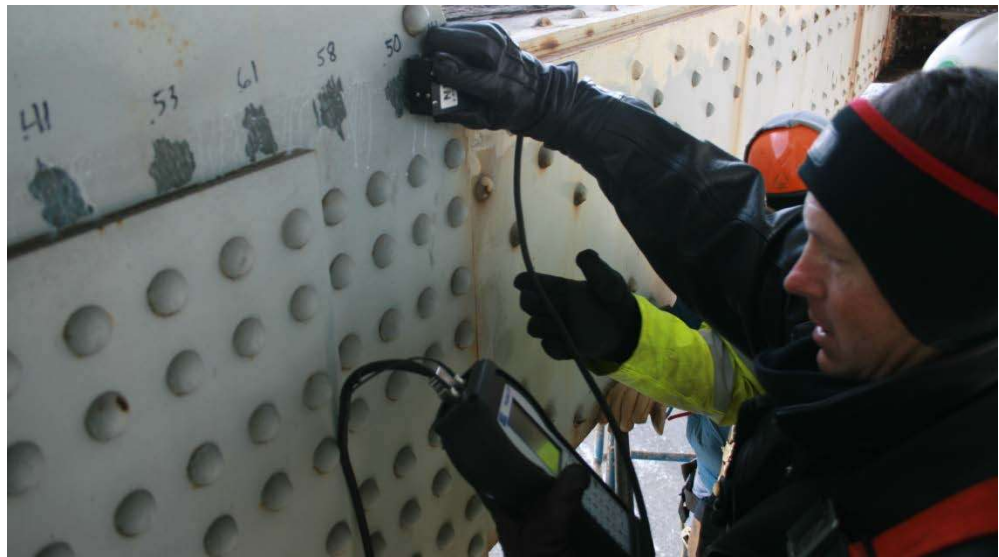
Figure 10.8.23 Inspector Using a Portable Ultrasonic Testing Inspection System
