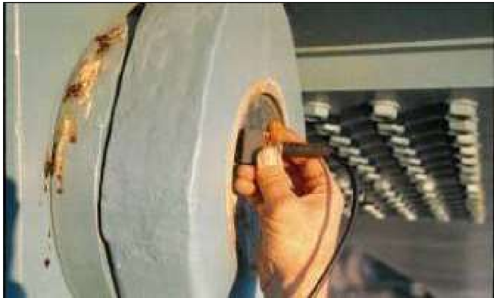
Figure 10.9.30 Ultrasonic Inspection of Eyebar Pin
