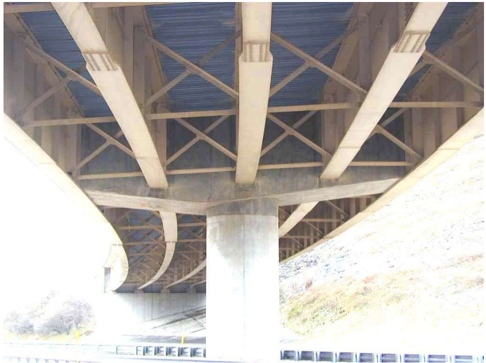
Figure 12.2.12 Integral Concrete Pier and Pier Cap
