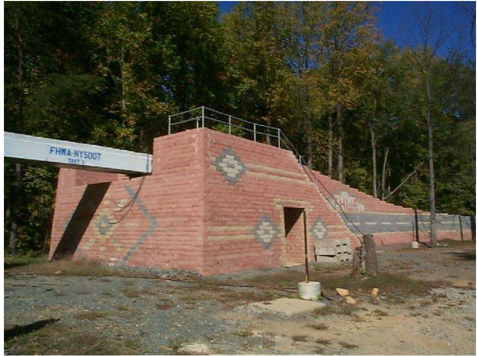
Figure 12.1.11 GRS Bridge Abutment at the FHWA Turner-Fairbank Highway Research Center
